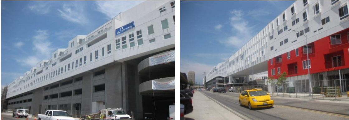
1st Santa Fe, Los Angeles. Michael Maltzan, architect.
