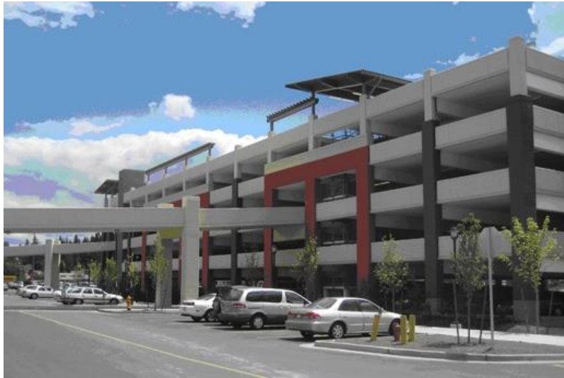
FIGURE 1 King County Metro Transit Parking Structure
